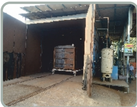
SHOT BLASTING BOOTH
